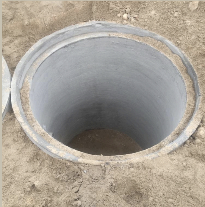
RCC water conservation
